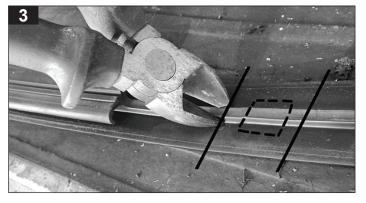
Turn roof ditch mould upside down. The underside rib has metal inside. Use side cutters to cut either side of hole position.
