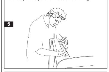
Marked out holes can now be drilled through using a 5mm drill bit and drill stop. Set the drill stop to ensure you don't drill through the roof lining. Use of a drill stop will alleviate the need to remove the hood lining.
